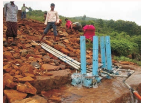
Hydraulic ram for upland irrigation
