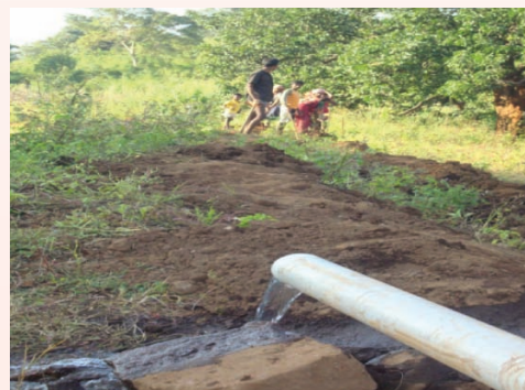
Ongoing buried pipe irrigation project
