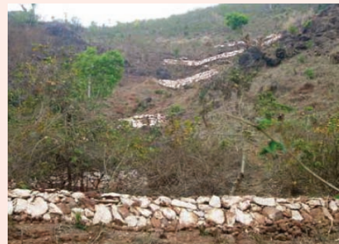
Loose boulder structure in series
