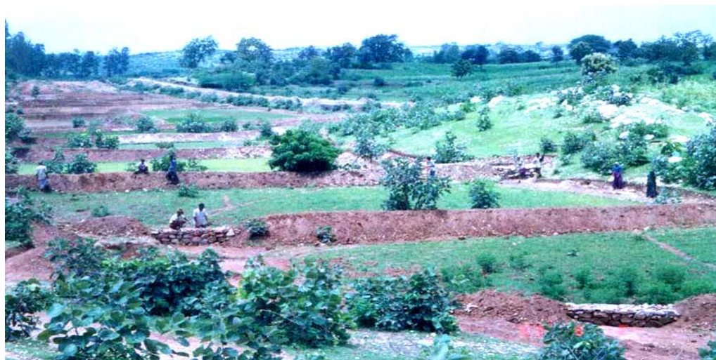
Fig. 5.3 Compartmental Bunding
