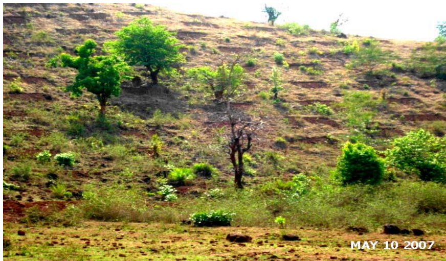
Fig. 5.7 Staggered Contour Trenches
