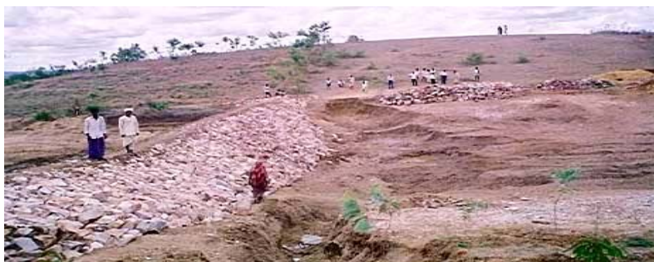
Fig. 5.41 Percolation Tank under Construction
