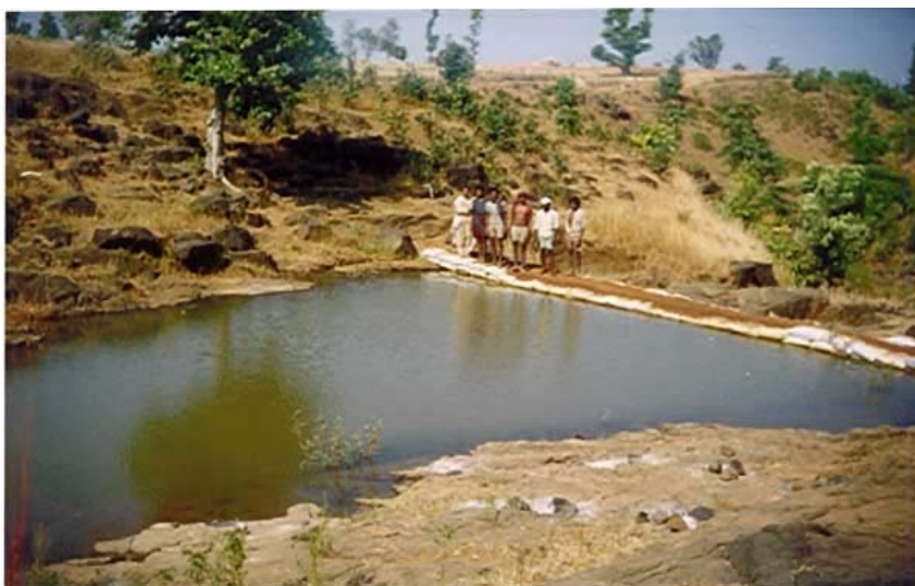
Fig.5.34 Water Harvesting Structure
