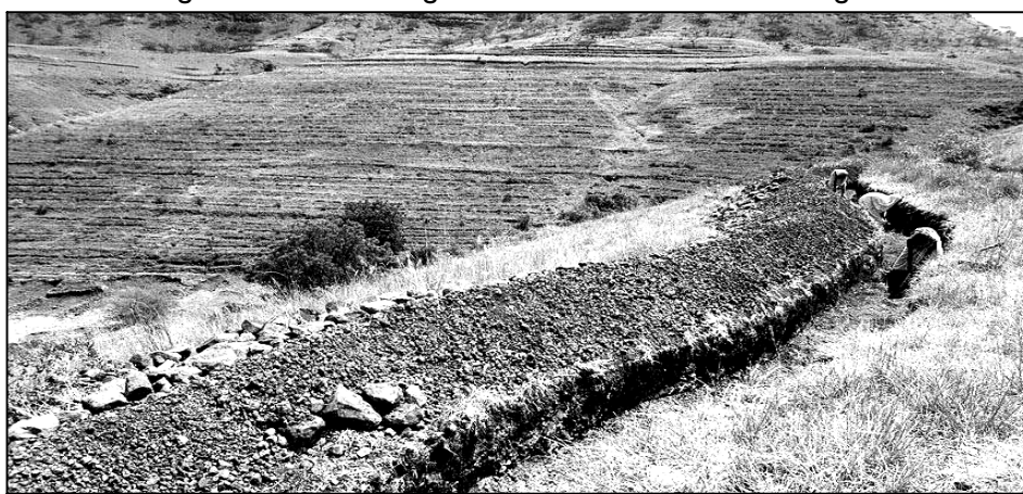
Fig. 5.8 Water Absorption Trench
