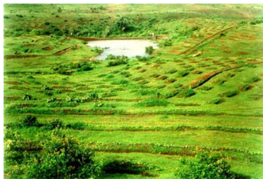
Fig.5.10 Combination of WAT & Staggered Trench
