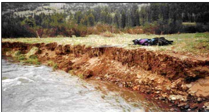
Fig.2.5 Stream bank erosion
