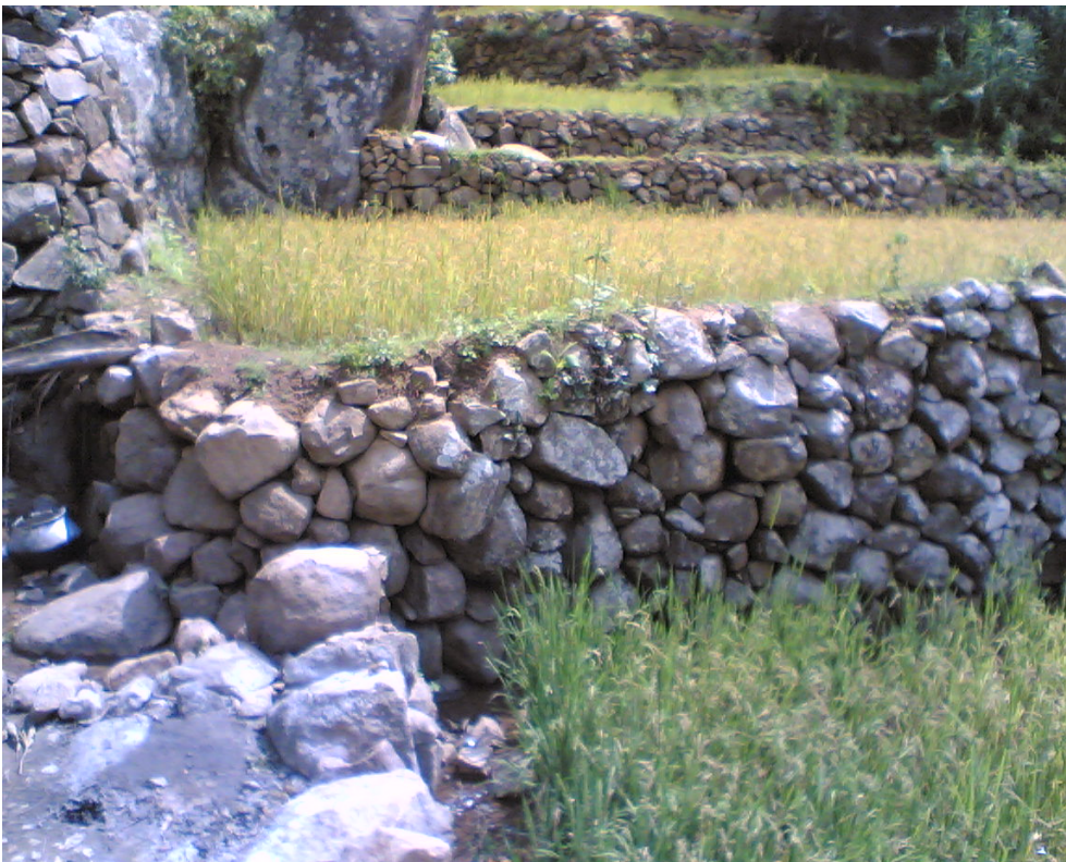
2. Stone Bunding for Field Cropping
