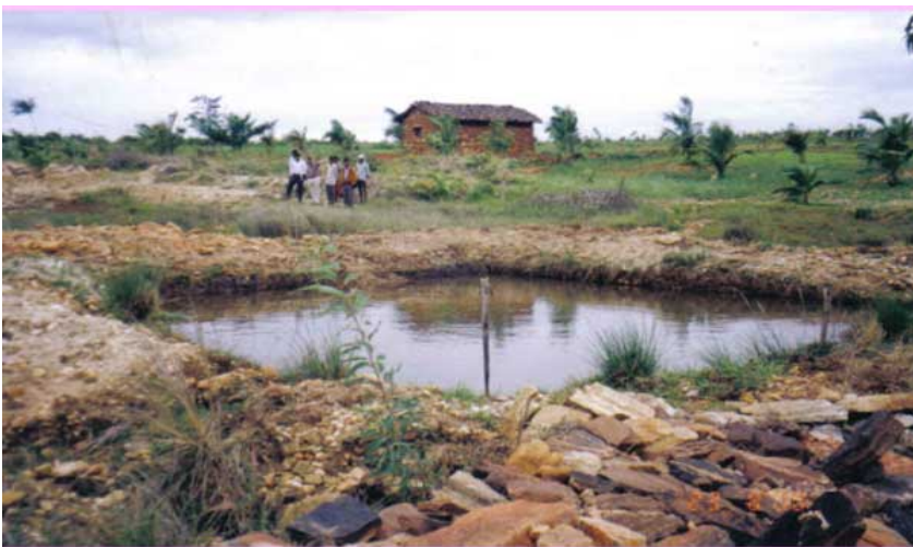
9. Water Harvesting Structure
